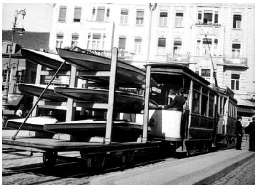
Bydgoszcz 1936, a special tram trailer transporting canoes to Brda.
