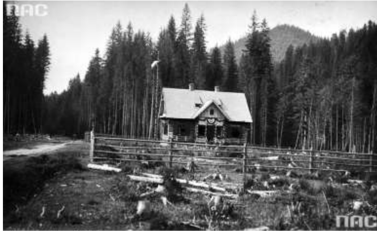
1926 View on the tourist hostel in the Jali Valley in Gorganach before ceremonial opening, photo: A. Siermontowski, NAC sets, ref. 1 - S-3739-2.
