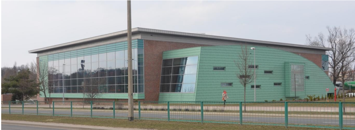
Fig.1. The University Swimming Pool in Olsztyn (source: photo M. Druszkowski 2013)
